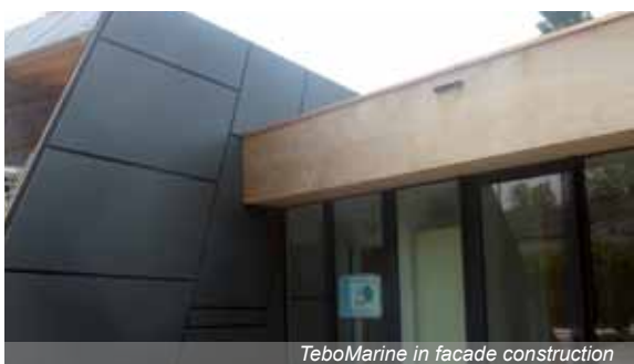
TeboMarine in facade construction
